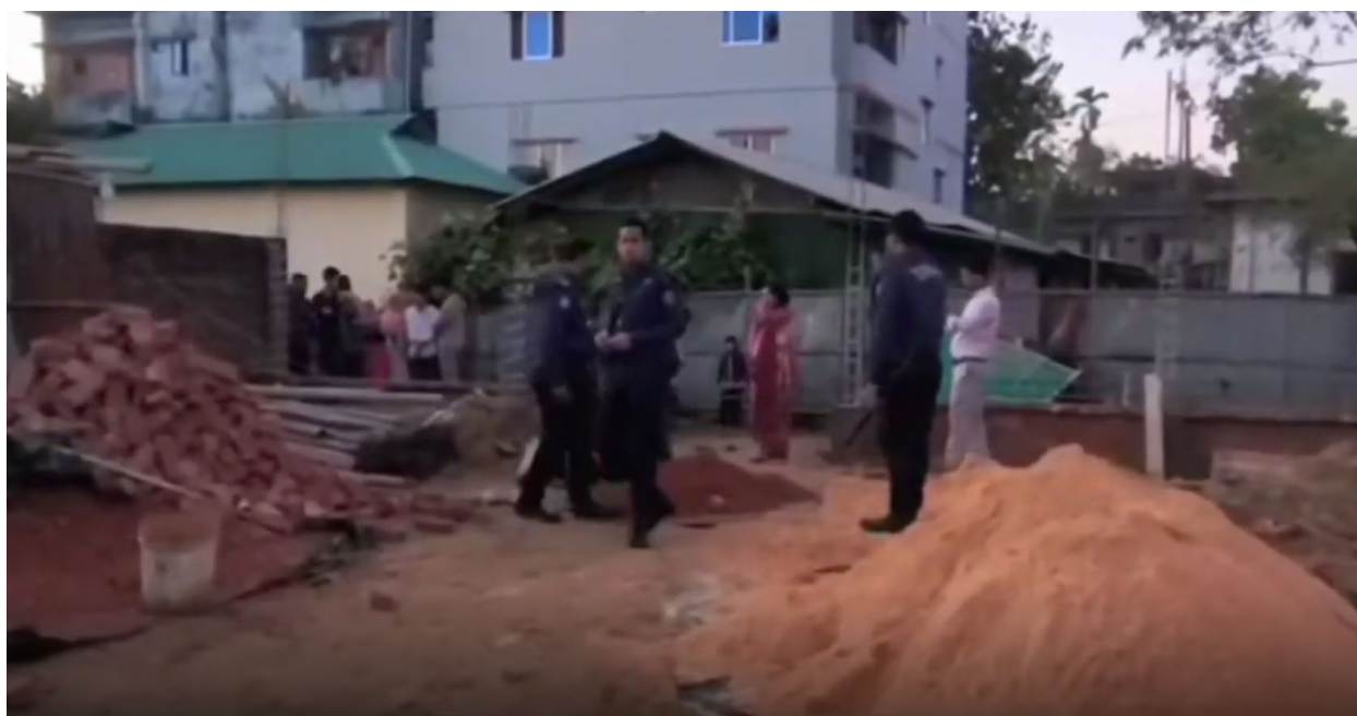
Figure 19. Attempted land grab targeting a Hindu family near a BGB camp in Cox's Bazar — video grab showing police inspecting the reported incident site after the attack. Four members of the minority family were reportedly injured while resisting the alleged forcible occupation of their land.
