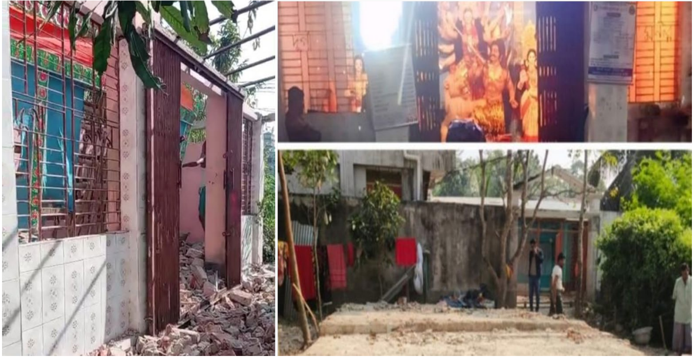
Figure 9. Demolition of historic Durga temple, Gournadi, Barishal — HRCBM SL 14.
